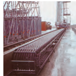
35 steel chains with supporting frame applied to De Icing's equipment at München airport (Germany).
