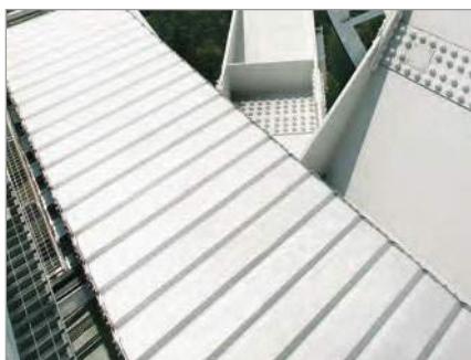
Steel cable carriers with aluminum cover system on a radio telescope Photographs: Max-Planck-Institut für Radioastronomie
