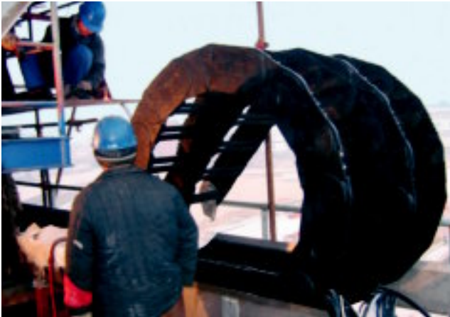
Assembling of an e-chain® Series 800 in an igus® steel guide trough
